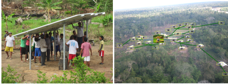
Smart solar micro-grid serves remote, isolated community (Bolivia)
